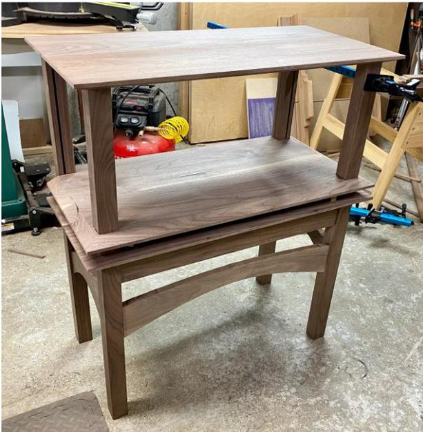
The photo to the left shows the construction of the case. The full height legs go through the two middle panels. The aprons and curved pieces at the bottom have traditional mortise and tenon joints to the legs. I cut the tapered edges on the top and two panels on the table saw and smoothed them out with a low angle jack plane and smoothing plane.
