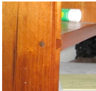
Square peg and sliding dovetail
