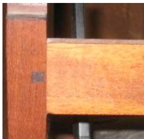
Square peg locking a tenon on the back of a bookshelf.
